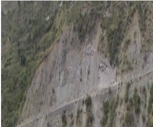
Photograph-7 Landslide of Baldogi
